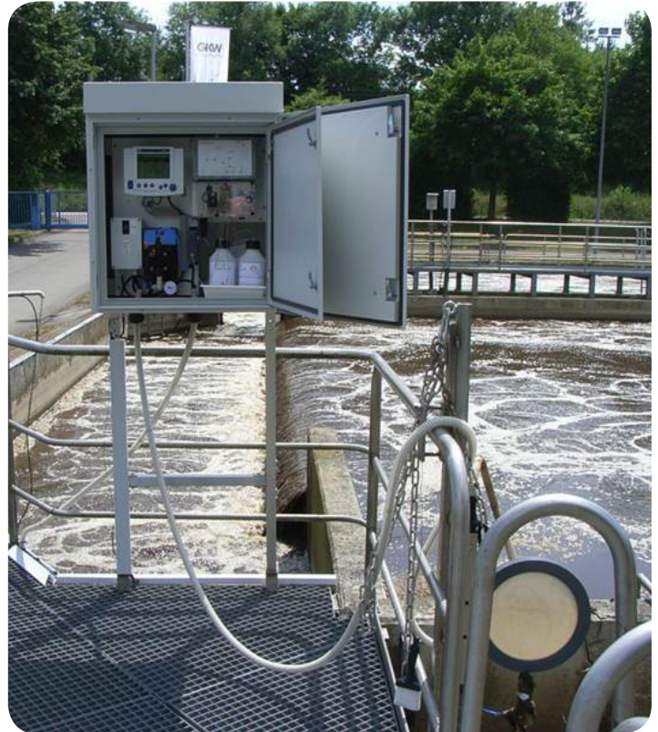
The YSI orthophosphate analyzer mounted outdoors next to aeration basin with the filter shown in the foreground.
