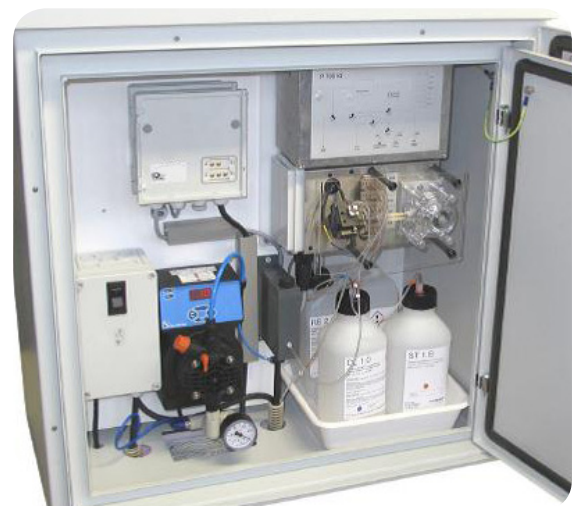
Inside view of the YSI orthophosphate analyzer.
